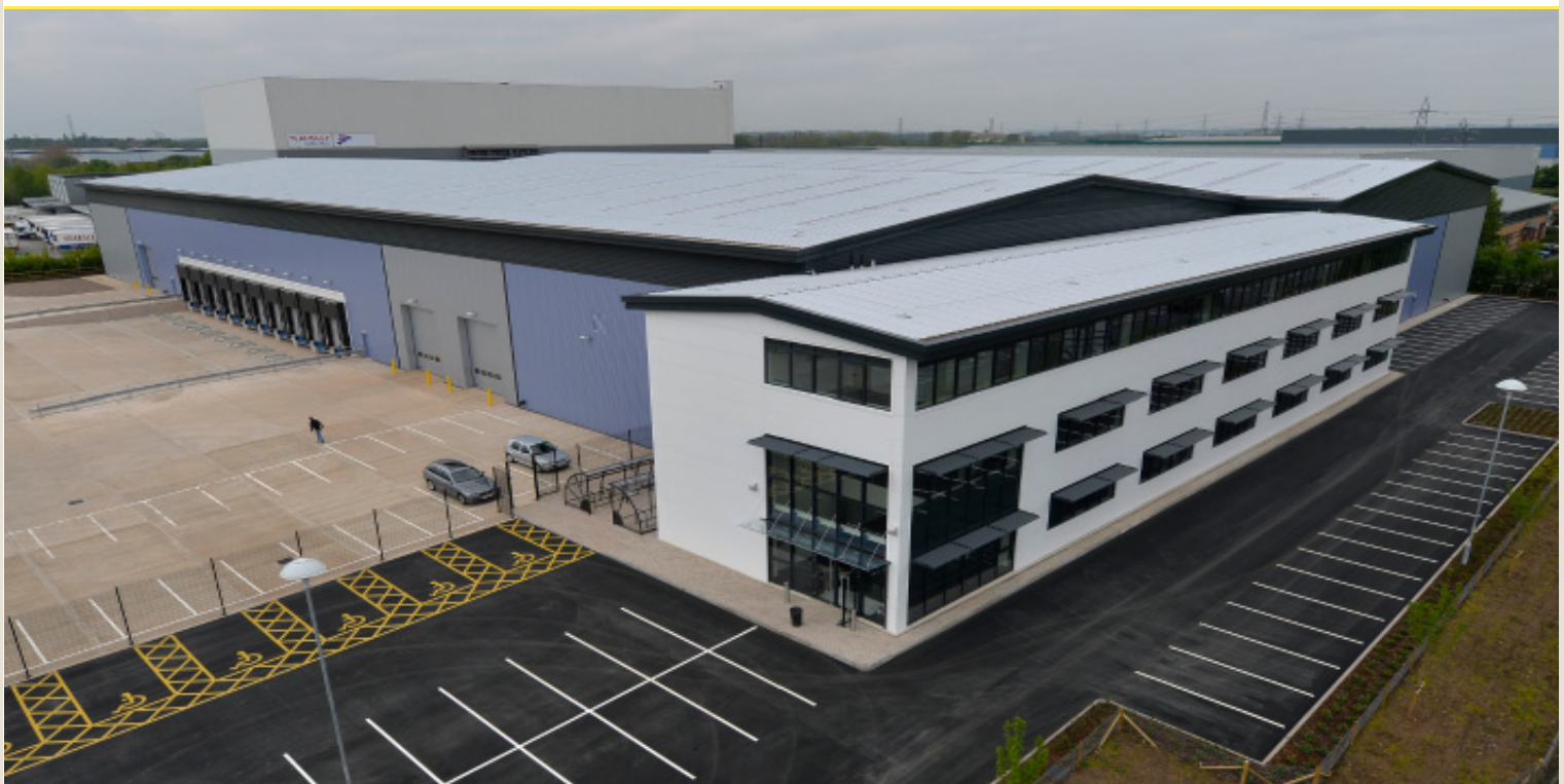
Silver Bullet at Hams Hall where Savills are marketing a speculatively built unit of 144,996 sq ft
